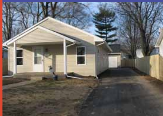
Finished! This home, like most of Habitat Huron Valley's is 40% more energy efficient than a typical new build.
